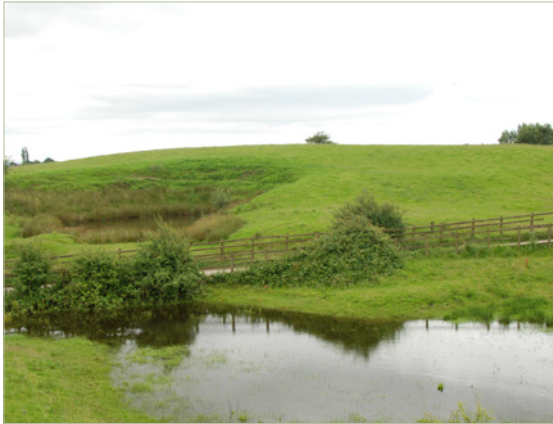
Undulating landform and ponds within the site
